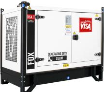
MAIN DATA Continuous power (PRP) kVA 13.70 Continuous power (PRP) 10.96 kW Emergency power (E.P.) kVA 15.10 Emergency power (E.P.) 12.08 kW 380 - 50 - 0.8 VAC - HZ - cos(fi)
